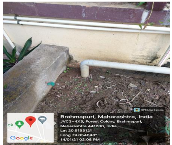
Soak pit for Hazardous Chemicals
