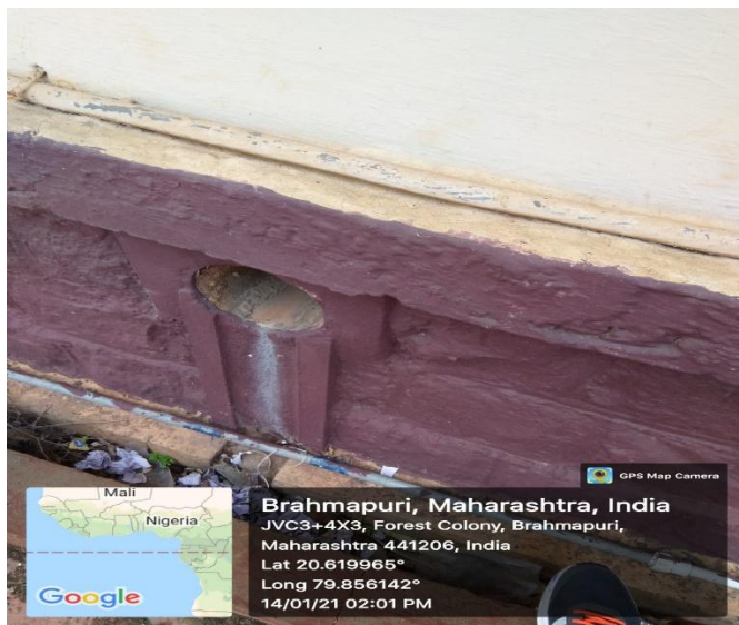
Sewage Line for Laboratory Waste
