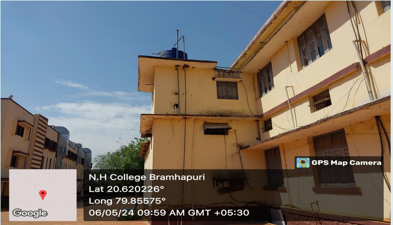
Water Distribution System in the campus
