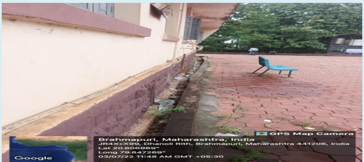
Soak pit and Canals for laboratory waste water Management
