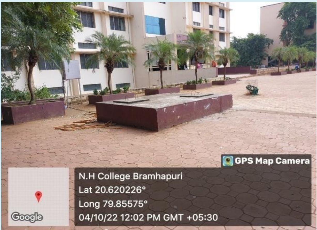
Water Storage Tanks
