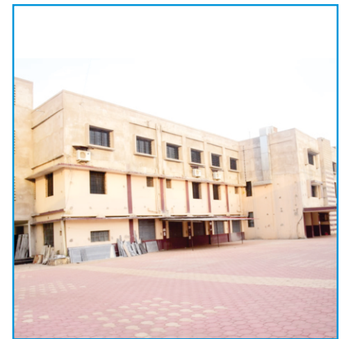
Central Library and Late Madangopalji Bhaiya Memorial Hall
