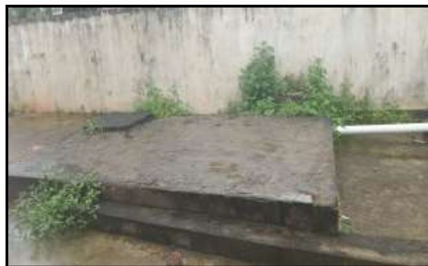
SOAK PIT NEAR BOYS HOSTEL
