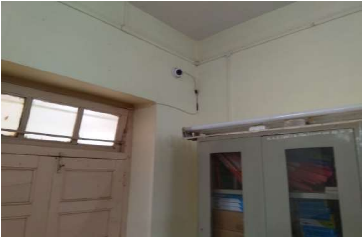
CCTV Camera in Laboratory
