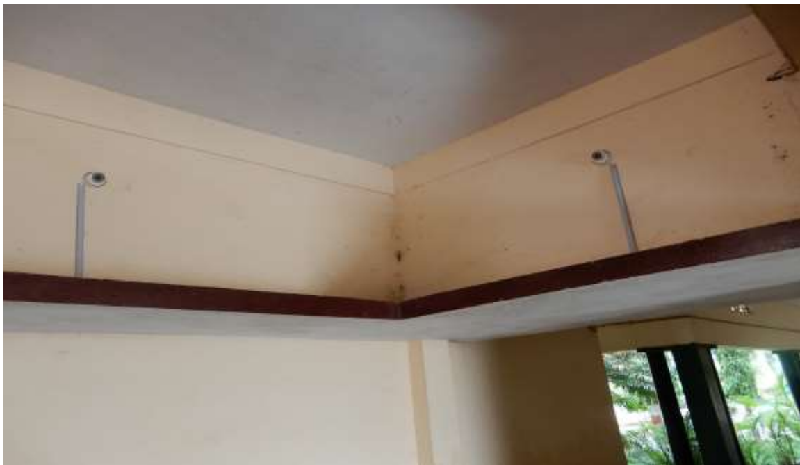
CCTV Camera in Corridor
