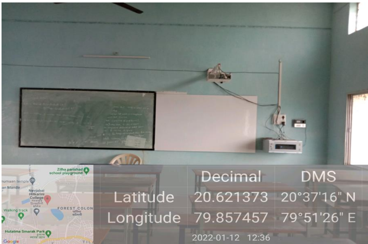
12. G-05 (Smart Class Room) (New Building)
