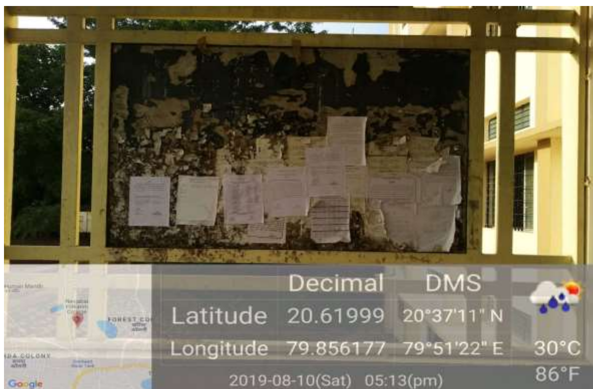
Notice Board at the front gate of PG Building
