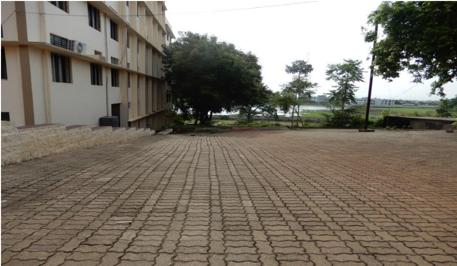
Slope for Rain Water toward Lake
